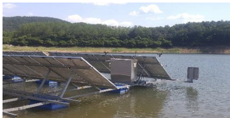
Fig.9 floating PV system in Soyang-river
