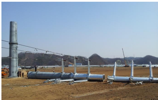
Fig. 1 Failure of pipe-type transmission tower
